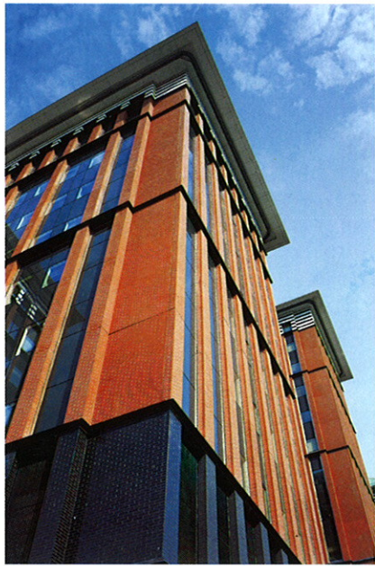
Cover picture: Reddish-brown clinker bricks in the facade and black ceramic clinkers in the plinth, besides the light and anthracite-grey granite, large window areas and black shaded glass panels are the specific design elements of the "Queens Tower", which the Architecture Photo describes in greater detail.
